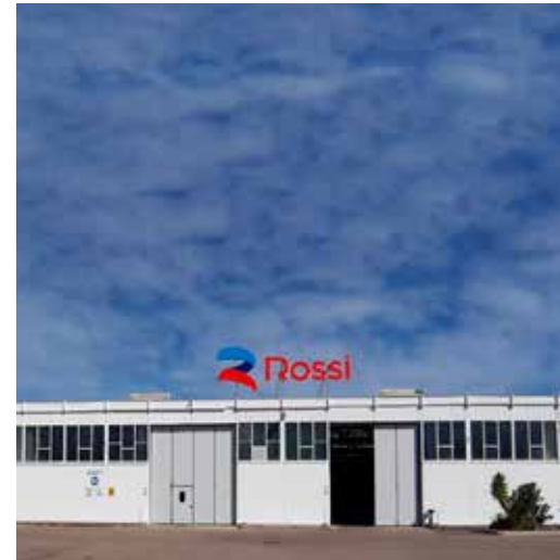
Planetary Division facilities Lecce - Italy
