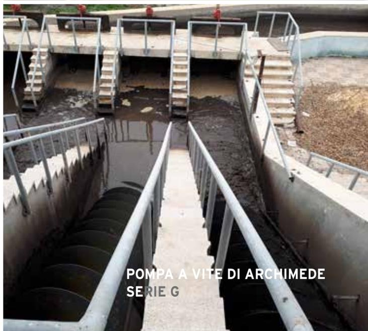
POMPA A VITE DI ARCHIMEDE
